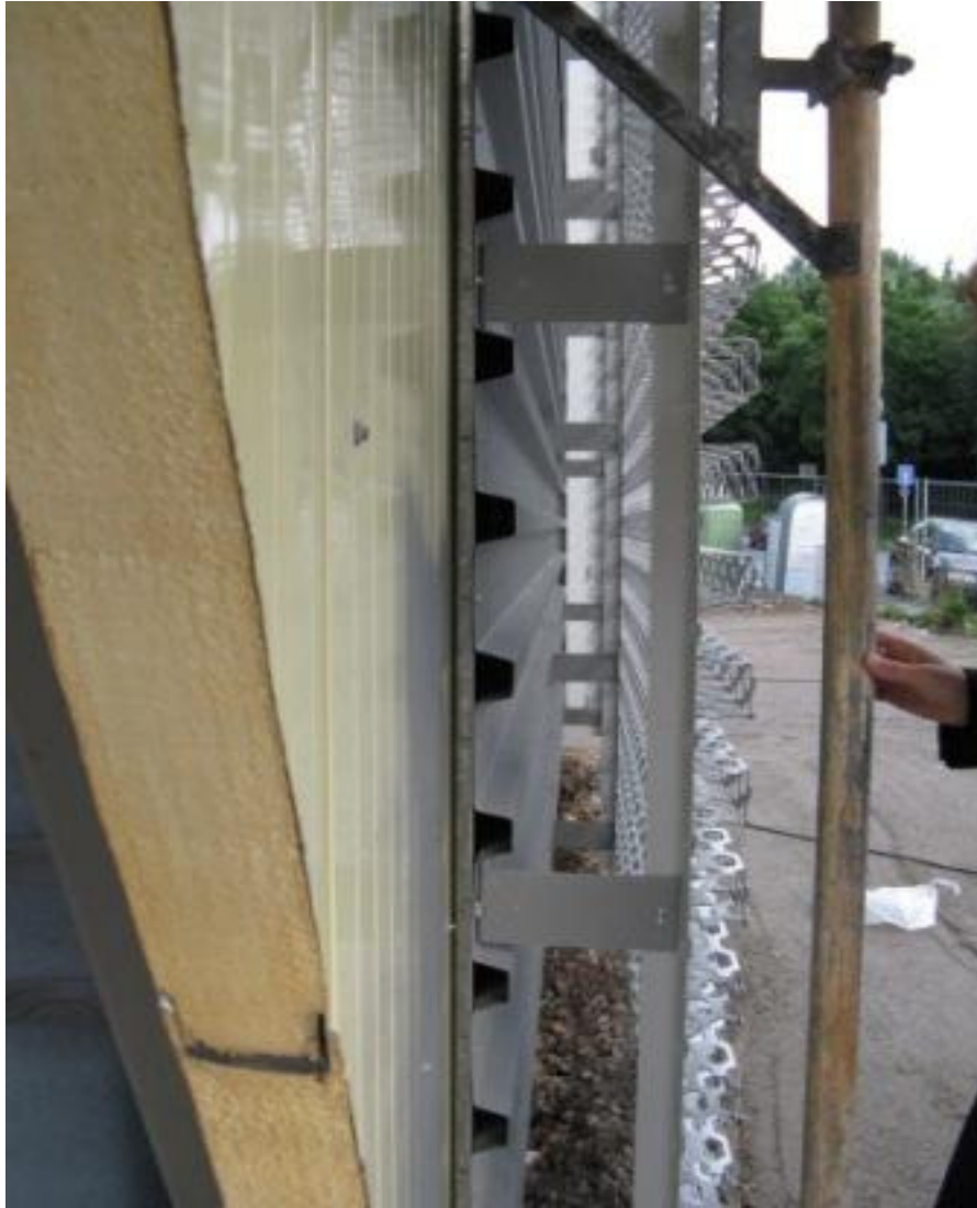
Example: detailed view of substructure with screwed aluminium profile angles + horizontal angles onto the bottom plate of the facade In this case: simple screwing between the corrugations of the trapezoidal sheet Screwing of the perforated panels onto the aluminium profiles.
