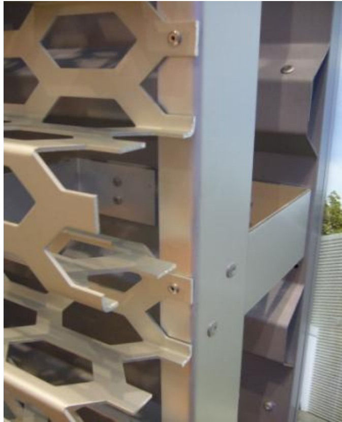
Example: Riveting of aluminium profile to horizontal angle + riveting of horizontal angle to trapezoidal sheet of facade Riveting on facade done between the corrugations. Afterwards riveting of perforated sheet on aluminium profile.
