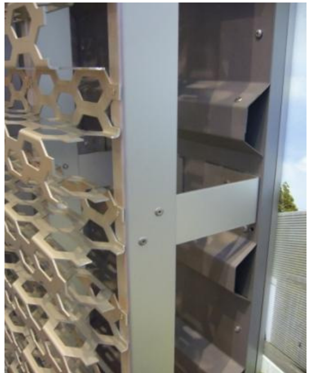
Example: Riveting of aluminium profile to horizontal angle + riveting of horizontal angle to trapezoidal sheet of facade Riveting on facade done between the corrugations. Afterwards riveting of perforated sheet on aluminium profile.
